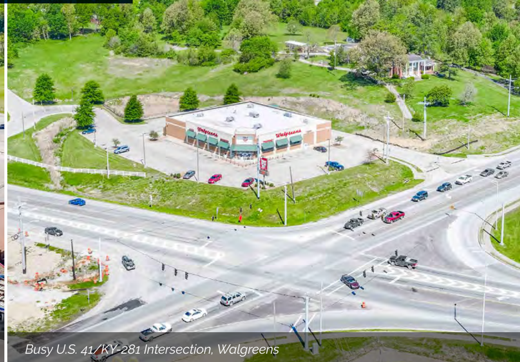
Neighboring Multi-Tenant Retail Center Includes Safeway Grocery & Dollar General
