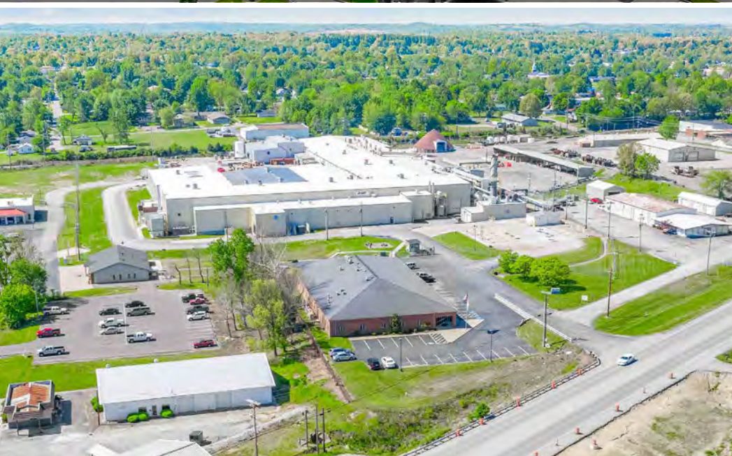
Adjacent Distribution Center and Major Employer, New Road Construction
